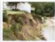
Human-managed streambank can lead to stream bank erosion. This can affect stream quality and habitat and cause property damage. Photo: Pennsylvania DEP
