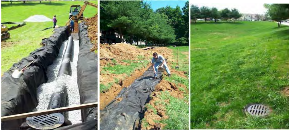
Figure 3: Example of Infiltration Trench Installation
